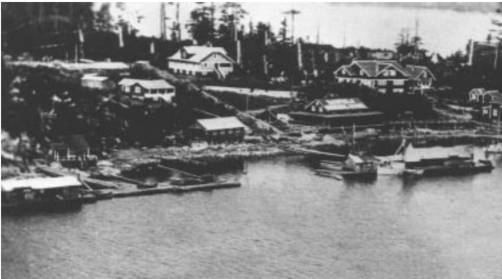
Bamfield in 1932, looking west across the inlet from the cable station to Aguilar Point. The large float just left of centre is my father's; to its left on the shore sits his net shed. Just up the hill from that you can see the Wickham residence, and to its right Uncle Charlie's hotel. Right of that is the large post office building,
